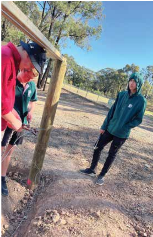
Phil Carroll Archer, Will and Nasa work on straining up the support wires on the chook shed fence.
