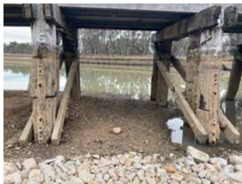
Restoration in process.
