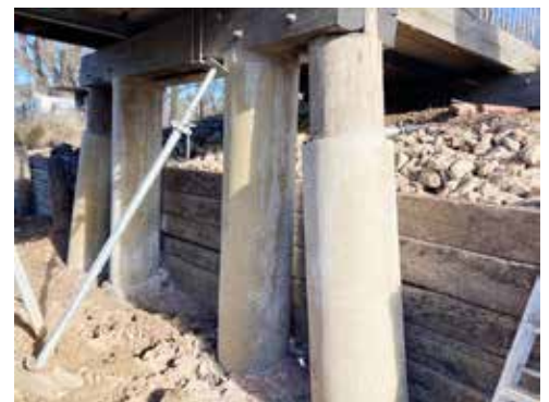
Pier repaired and drying
