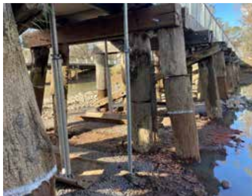
New pier foundations underway.
