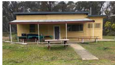
After the clean-up and paint.
