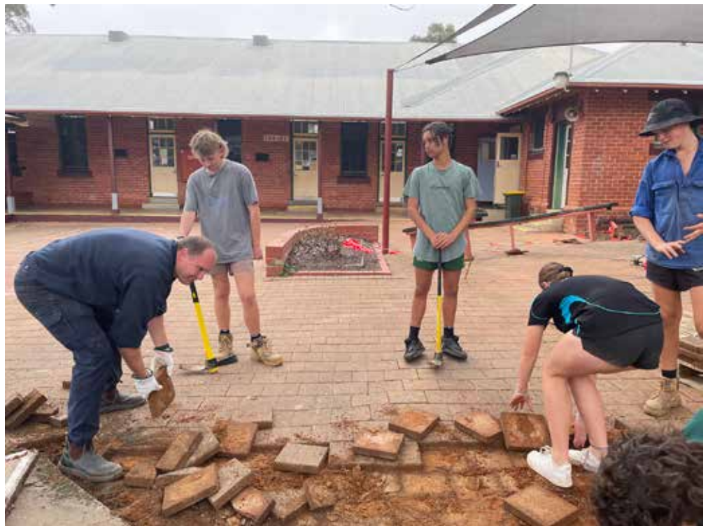
Lifting the pavers under the shade sail area.
