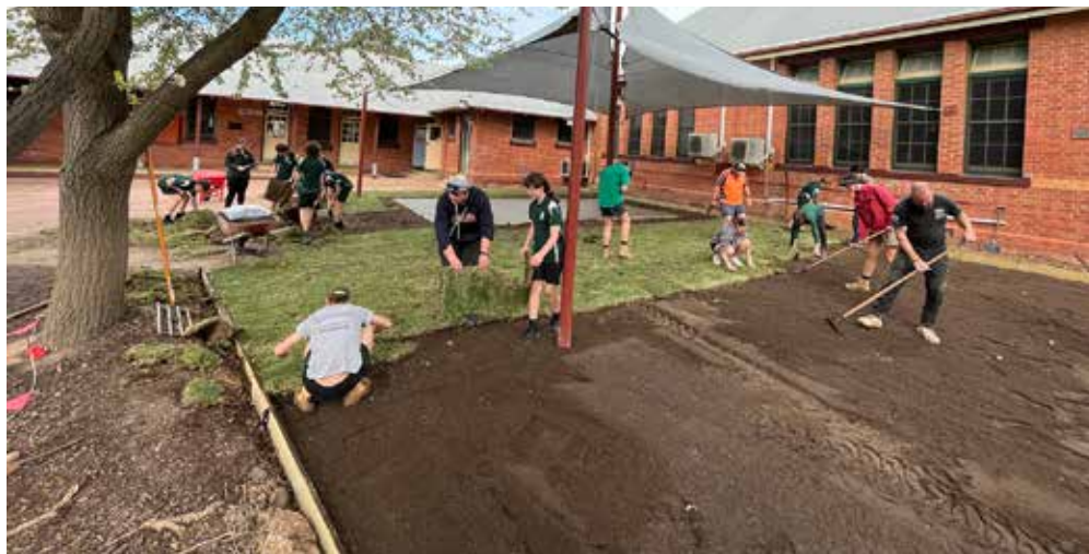
Spreading the soil for some new turf, everyone working hard.
