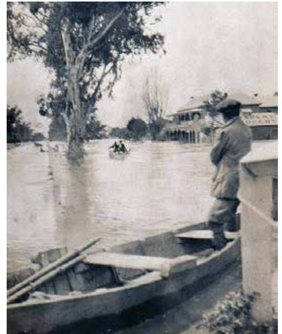
High Road Murchison-east, off the bridge 1916
