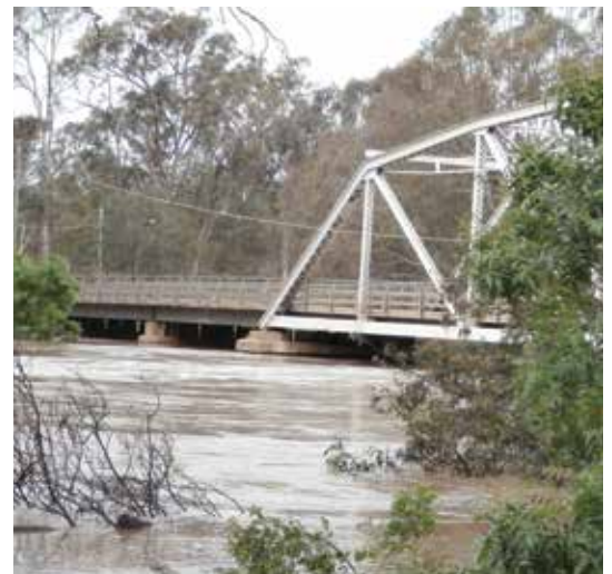
River level under the bridge 15 October, 2022
